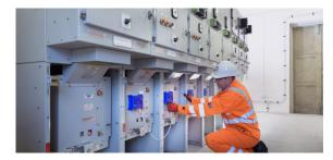
The **Astute® HV Monitor** is part of the award-winning **UltraTEV®** range. It is an advanced asset monitoring system for 24/7 monitoring of PD activity in all substation electrical assets. The **Astute® HV Monitor** is a modular system with up to 300 sensors that can be located across a switchboard to offer optimised coverage – typically without an outage being required.
